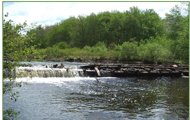
Remnants of Brunswick Mill Dam # 1. This dam was constructed of timber and rock.
